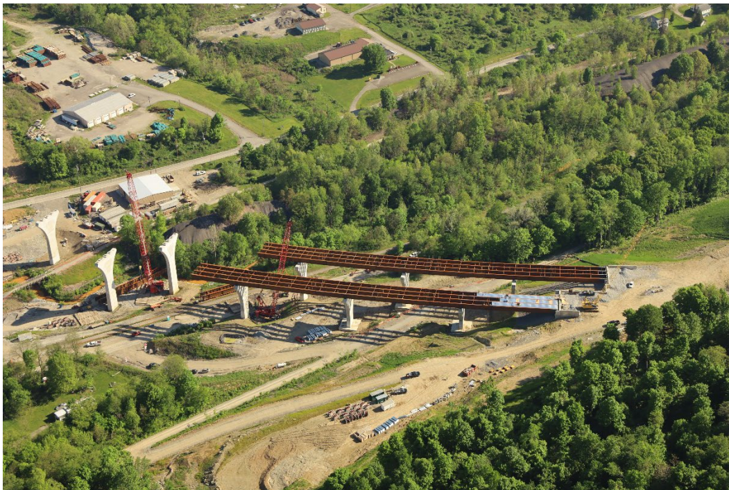
Photo 2 - Beam Erection
