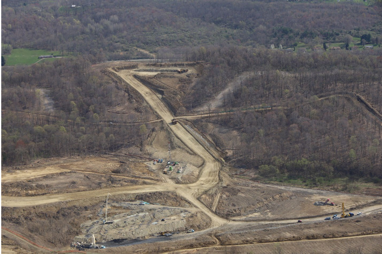
Photo 3 – Gas Well Plugging
