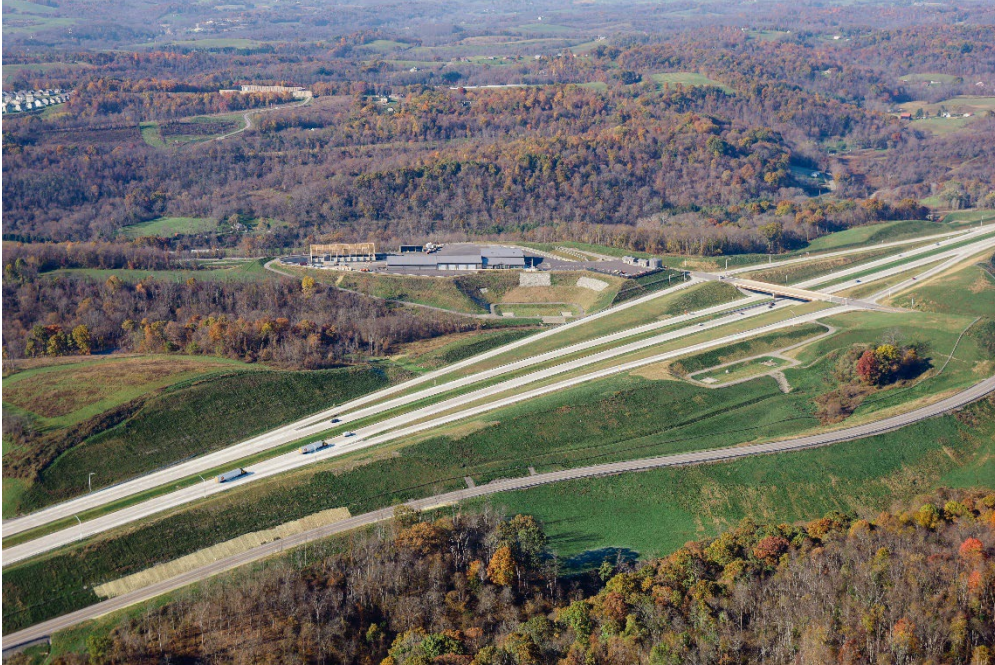
Photo 4 – Aerial View of Completed Interchange and Maintenance Facility
