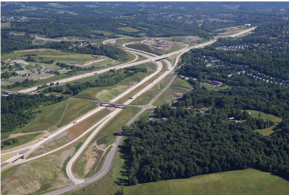
Photo 5 – Aerial View of Completed Interchange with I-79 and Morganza Road
